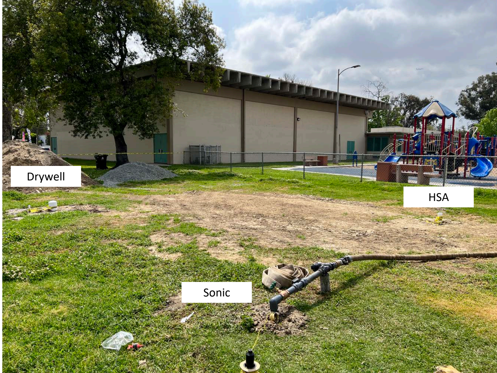
All three installations at Mary Bethune Park
