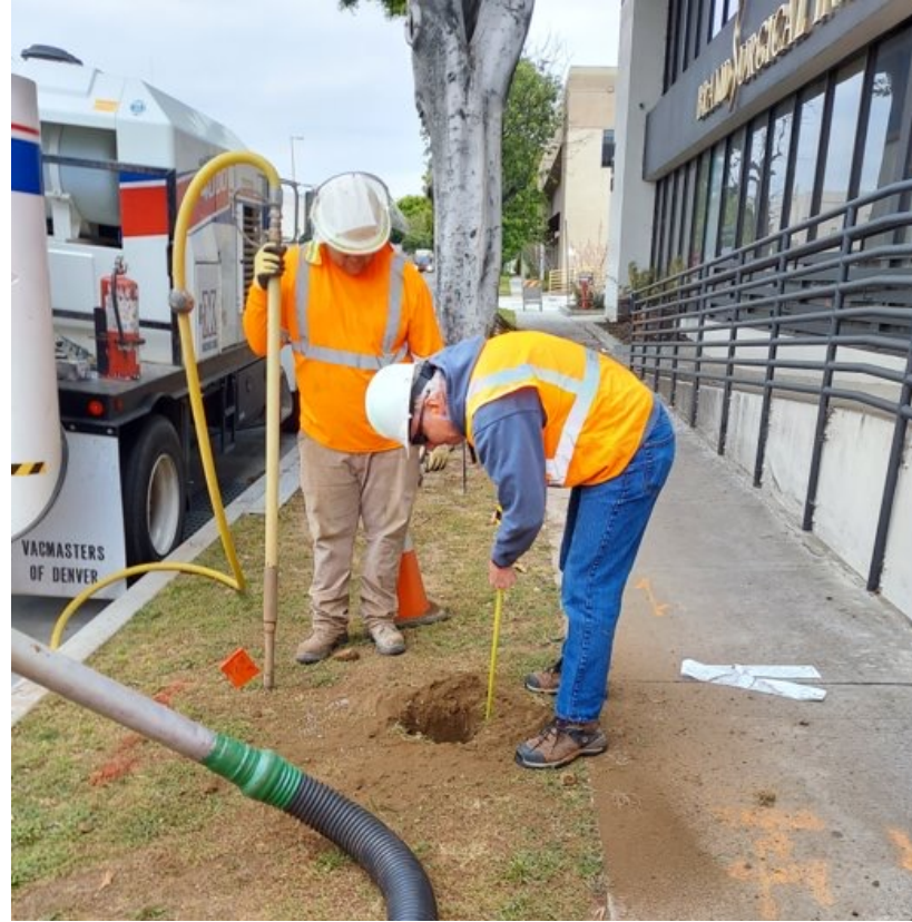
All well locations were potholed using vac-truck
