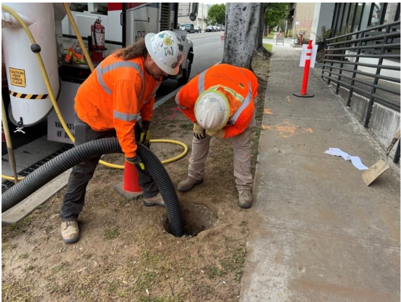
All well locations were potholed using vac-truck
