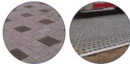
Permeable Pavement typ max slope = 5%
