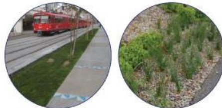
Vegetated Filter Strip typ max slope = 6-33%
