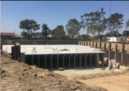
**Pre-Cast Subsurface Infiltration Facility**
