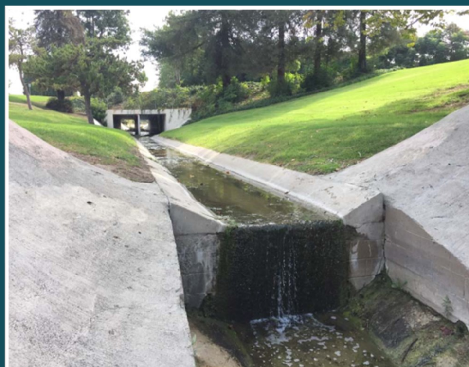
Existing Concrete Channel
