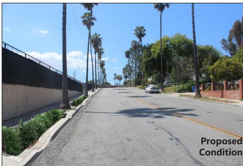
Parkway bioretention cells are proposed to capture and treat surface stormwater runoff along the public right-of-way. A total of **1,800 sq-ft** of impervious surface will be removed and replaced with vegetated cover.
