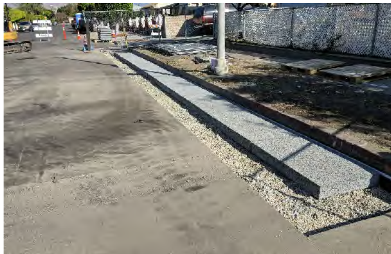
Figure 3-3 Construction of Pre-Cast Modular Concrete Gutter Slabs
