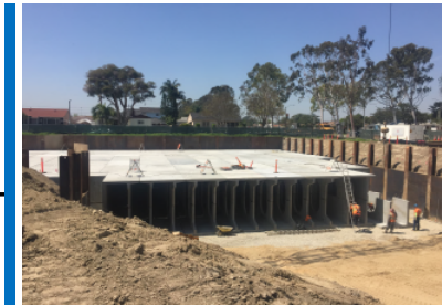
Pre-Cast Subsurface Infiltration Facility
