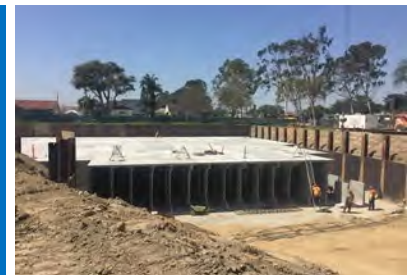
Pre-Cast Subsurface Infiltration Facility
