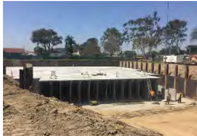
Pre-Cast Subsurface Infiltration Facility
