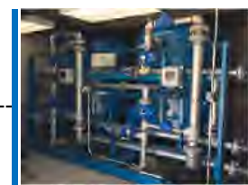
Stormwater Harvesting Unit
