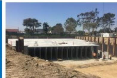
**Pre-Cast Subsurface Infiltration Facility**
