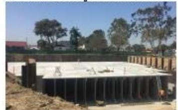
Precast Concrete Underground Infiltration Chambers
