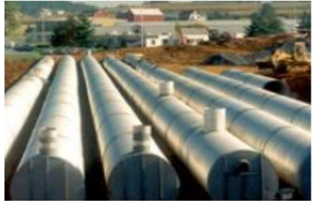
Corrugated Metal Pipe – infiltration galleys to be located under the field turf
