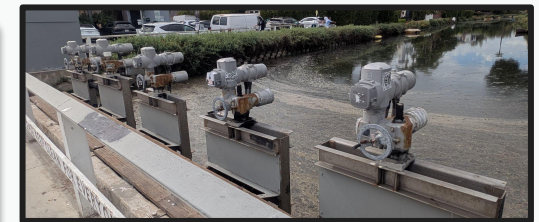
Existing Tidal Gates – Washington Boulevard
