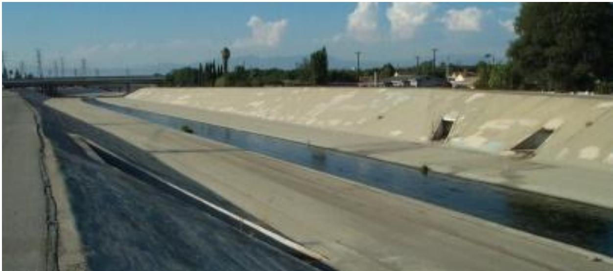
Figure 2-6. Looking down San Gabriel River's concrete-lined channel in the lower coastal plain
