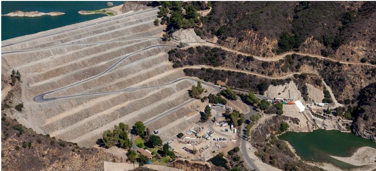
Figure 2-7. San Gabriel River Dam (LA County Department of Public Works)
