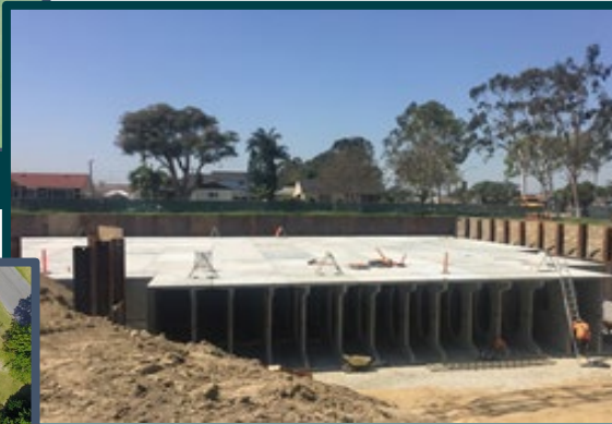
1.6 AC-FT UNDERGROUND INFILTRATION GALLERY
