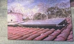
Hor water for this building is provided by a solar collector on the roof.
