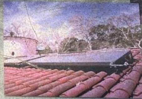
Hot water for this building is provided by a solar collector on the roof.
