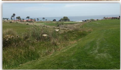
Existing drainage ditch converted to biofiltration swale with native grasses and sedges.
