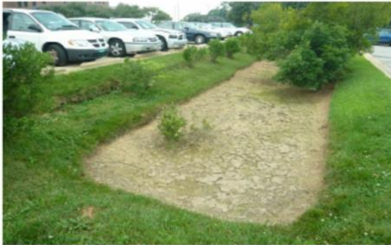
Clogged and eroding bioretention basins: Source (Blecken et. al, 2015)
