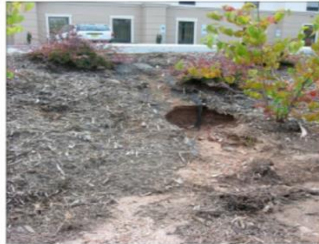
Clogged and eroding bioretention basins: Source (Blecken et. al, 2015)
